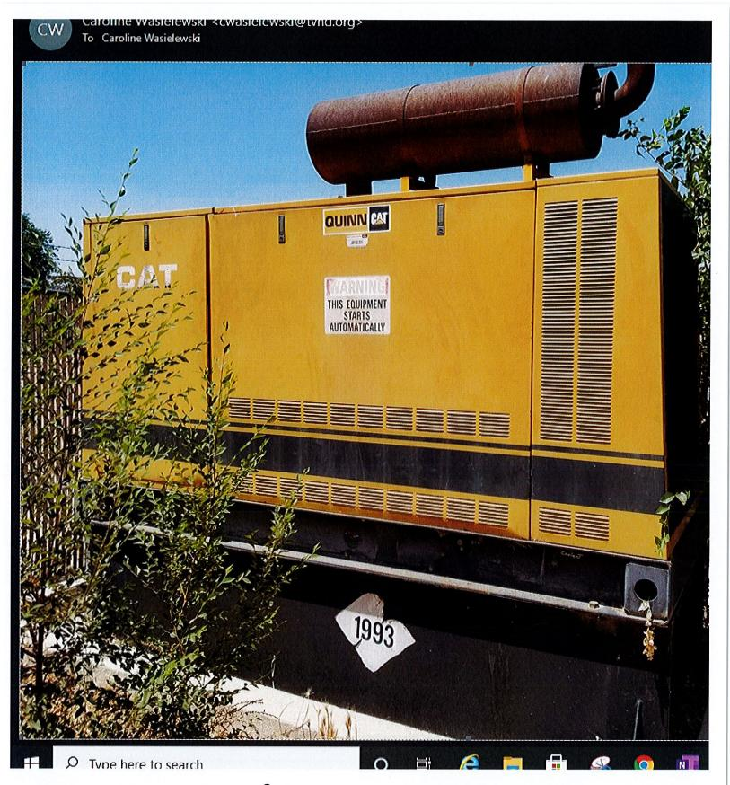
One 268 the Caterpillar Model 3208 emergency use piston organie powering 200kW electrical generator. Packet Page #10
